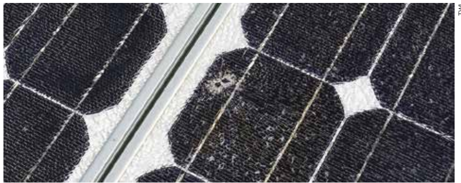
Microcracks can eventually cause an entire panel to shatter
